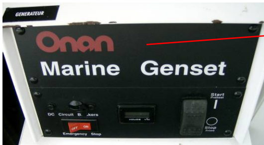
Main breakers for the generator
